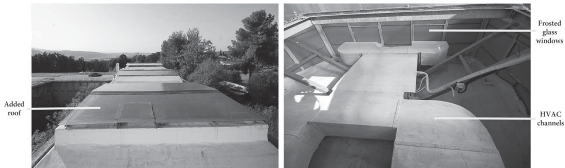
Figure 3. The gallery roof system today: polycarbonate lightweight roof (right), opaque windows and an air-conditioning system on the hyperbolic lightweight roof (left).
